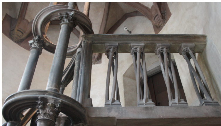
FIGURE 4. Villarceau circles and skew lines at Musée de l'Oeuvre Notre-Dame, Strasbourg, a photograph by Luba Shenderova-Fock.
